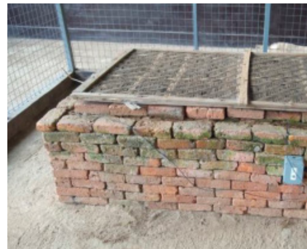
A brick Evaporative Cooling Chamber (with performance monitoring sensor attached), Rubona, Rwanda.
