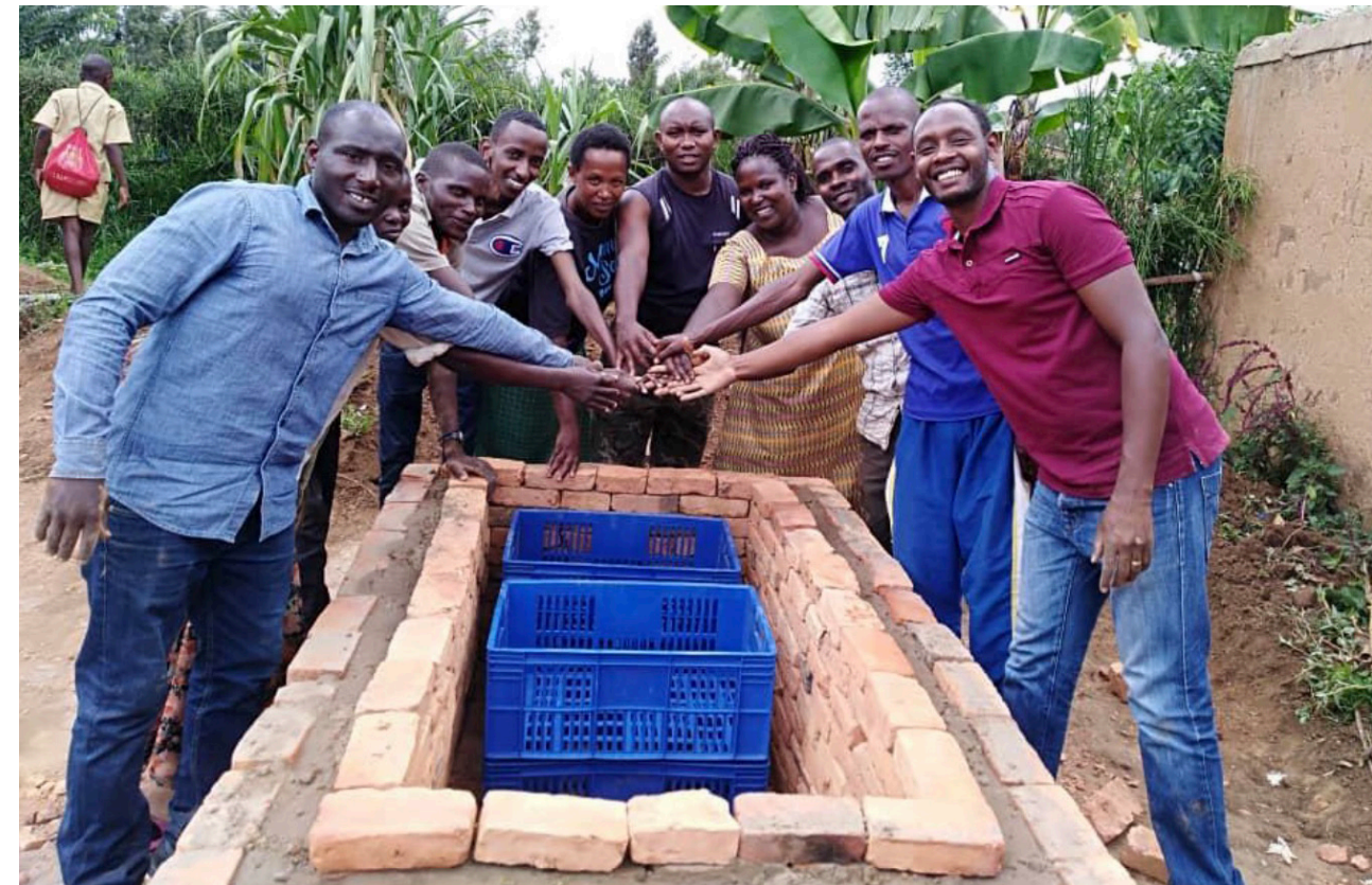
A completed brick Zero Energy Cooling Chamber in Gatisbo, Rwanda.
