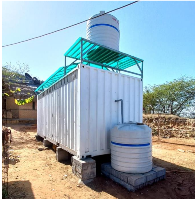
Figure 11: The rear of the pilot forced-air evaporative cooling chamber in Gujarat, India, showing the two water storage tanks.
