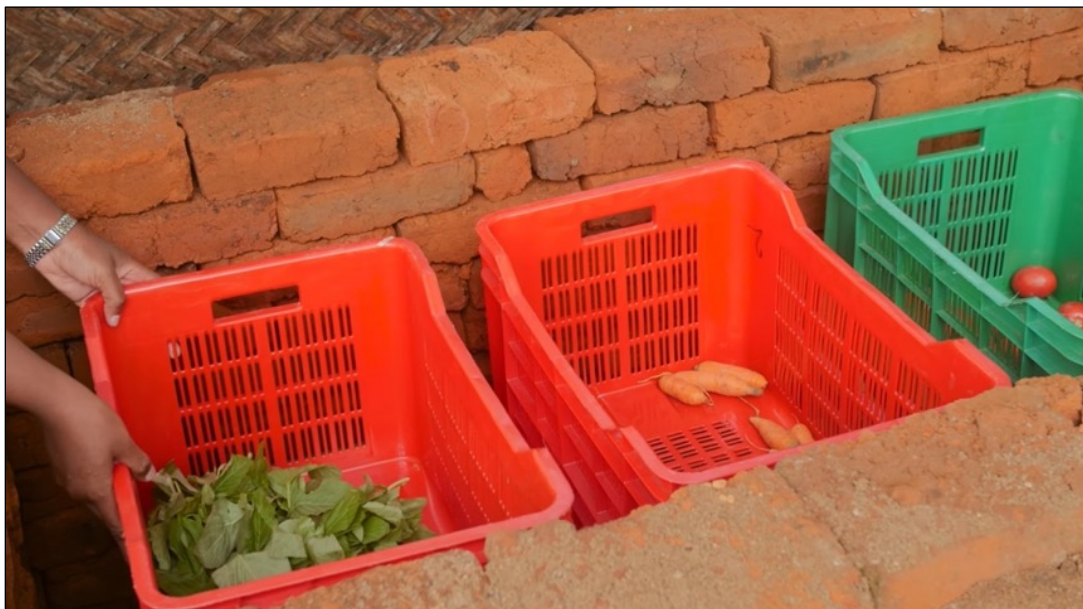
Vegetables stored in an evaporative cooling chamber
